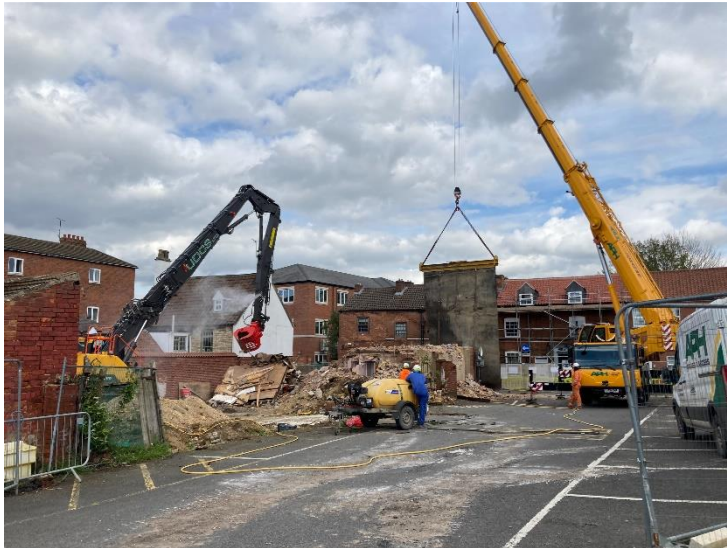
Figure 1- Demolition at Swinegate, a curtain was used to stop debris on the road so that it could remain open
